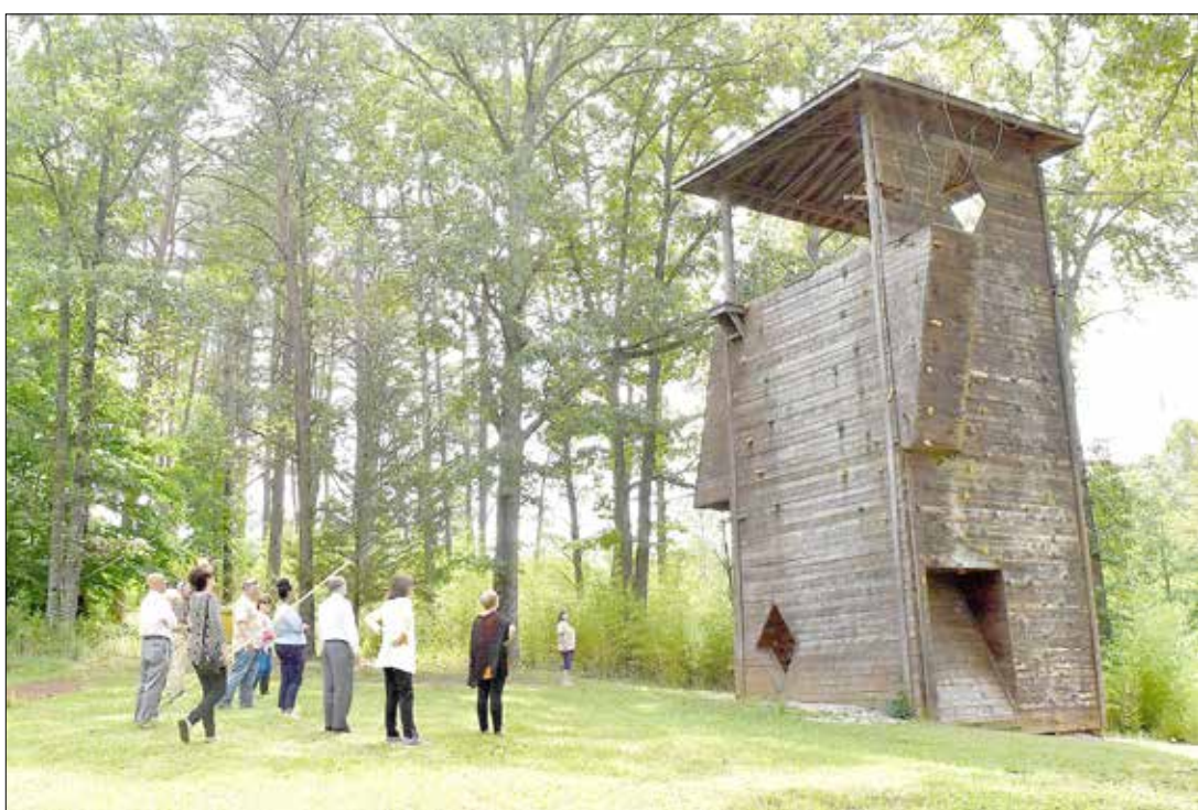
This is the climbing tower and high ropes course at Lee Ford Camp. Repairs are needed to the ropes course's cable connections on trees.
