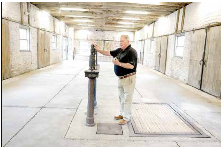
A scale, believed to be original to the train depot, remains in the former cargo room of the depot. The original patina of the brick walls and wooden doors has been preserved.
