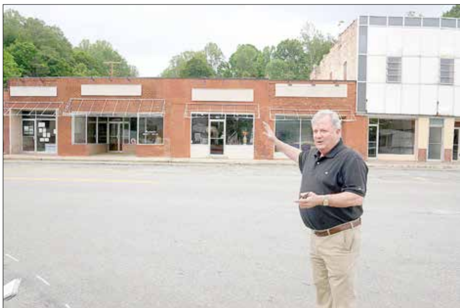
Renovations are planned for the facades of some of the storefronts on the Reed Stone Block adjacent to the depot.
