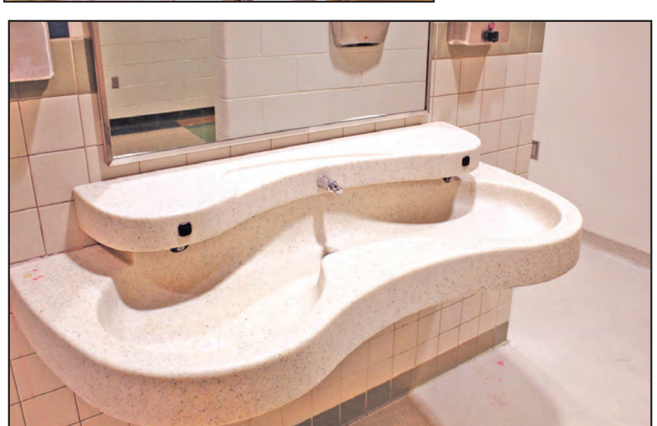
Meadow View features low-flow toilets, motion-activated sinks, and automatic water fountains to conserve water.
