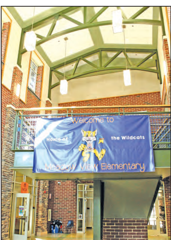
Meadow View Elementary School in Henry County was constructed intentionally with lots of windows and skylights to cut down on electric lighting costs. The glass is coated and features removable shades to prevent energy from escaping.
