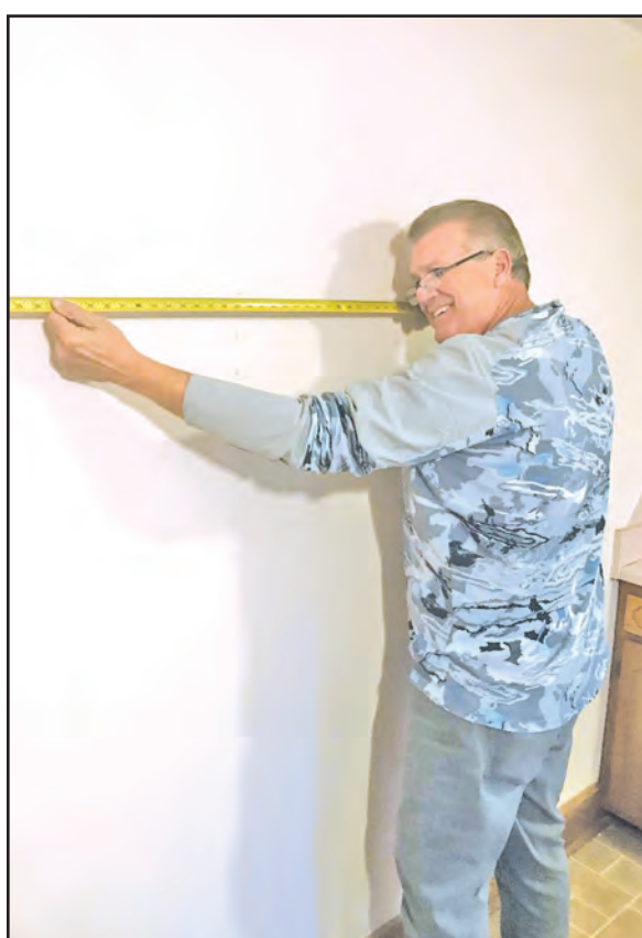
Board member John Collins takes measurements in preparation of appliance installation.
