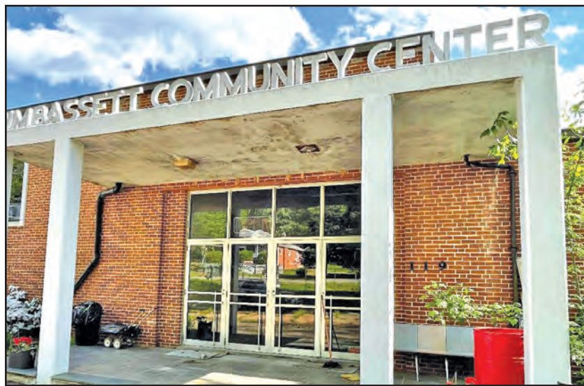
The W. M. Bassett Community Center on Blackberry Road is in a state of disrepair and disarray, but one group resolves to tackle the challenges and explore options to reopen the facility.
