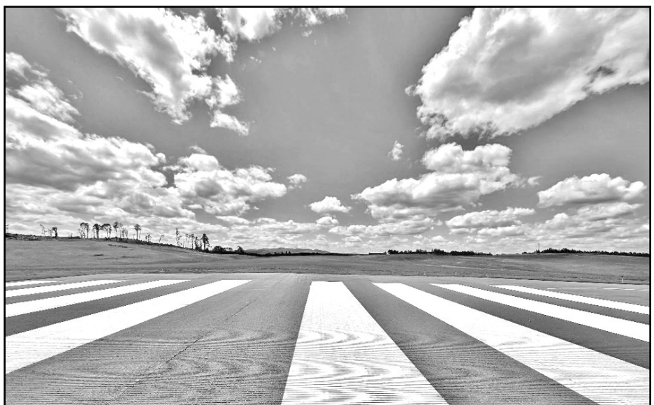
The Blue Ridge Regional Airport has a planned 1,000-foot runway extension. Pictured is the direction of the planned extension.
