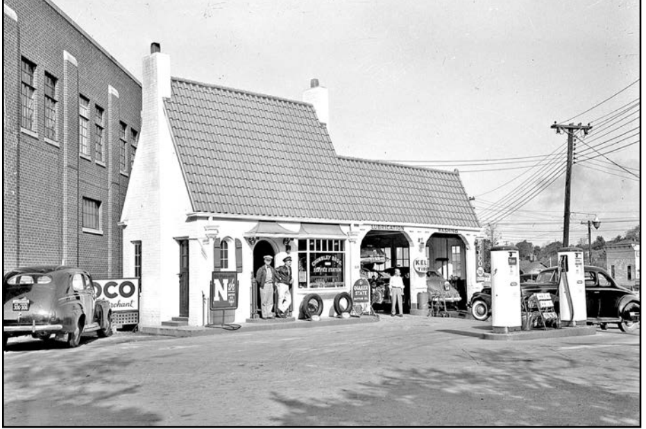
This Tudor Revival-style square station was built for the Proffitt brothers on the northwest corner of the service in Christiansburg during the early 1930s. The building was a standard company design built across the country after 1927. The Christiansburg station was operated by the Chumbley Brothers at the time of this 1948 photograph. (This image from the D. D. Lester Collection and many more are available from the Montgomery Museum of Art & History.)
