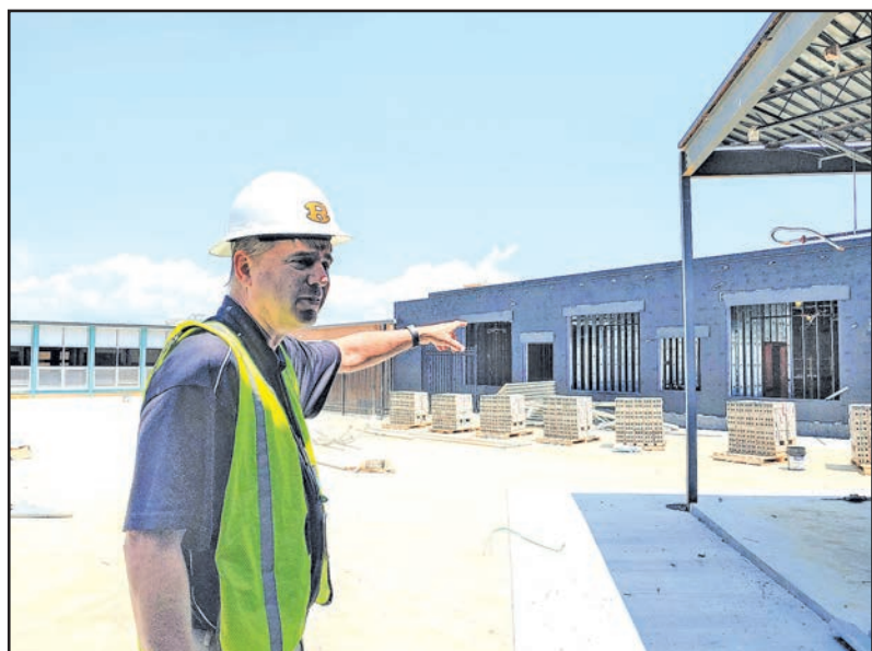
Radford Superintendent Robert Graham looks over the progress of the McHarg Elementary School renovation project Thursday.
