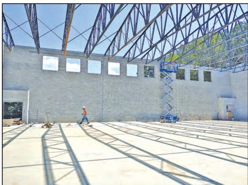
The large floor plan of the new gymnasium can be seen against the backdrop of the worker walking along the far wall of the structure.
