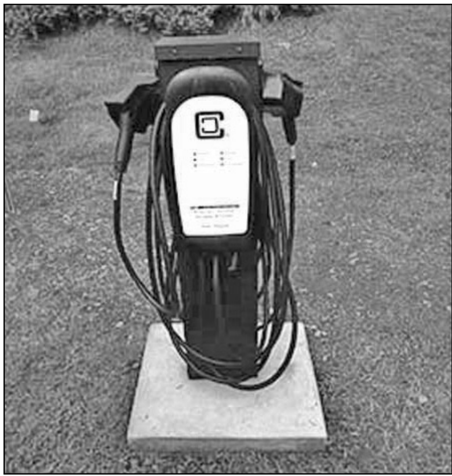
The electric charging station at the Montgomery County Government Center in Christiansburg has two charging ports, which allows two cars to charge at the same time.
