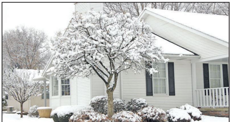
To prevent catastrophic damage to a home in the event of a sudden cold snap when the family is out of town, bump the thermostat into the 60s, not the 50s, let the faucets drip, and have a neighbor or friend check on the home periodically. Then remove any snow from the roof as soon as possible after returning home to prevent the snow from freezing.
