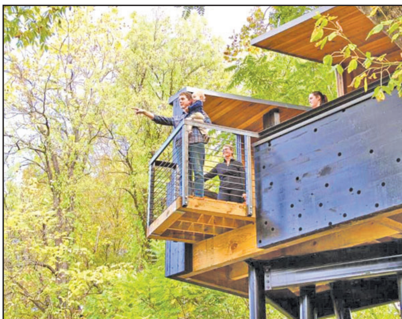
The observatory's designers are the recipients of a national architecture award for the project, located below Glencoe Mansion, Museum, and Gallery.
