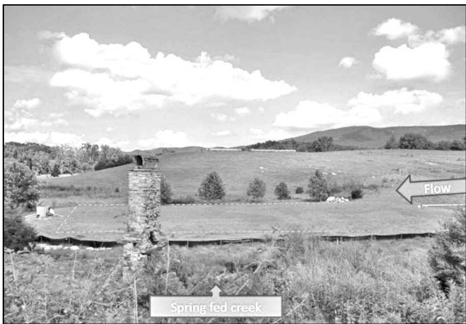
Pictured is a side view of the Shenandoah Valley spring bioreactor. The water inlet pipe is on the right, and the bioreactor is outlined by dotted line. Beneath the surface is 3 feet of wood chips. Photo illustration by Kurt Stephenson for Virginia Tech.
