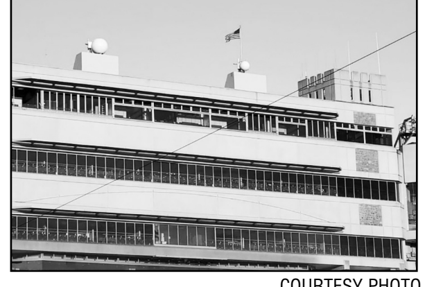
COURTESY PHOTO The new MatSing lenses were installed at Lane stadium in the fall, significantly improving cell service for Hokie fans during events.
