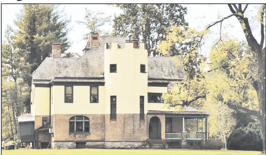
Built in 1892 by Captain "Billy" Williams Ingles along the New River in west end Radford, the architectural wonder is a Radford treasure.
