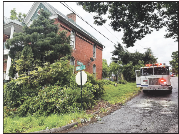
This home on Downey Street caught fire as a result of a downed power line. Firefighters were able to put out the fire quickly.
