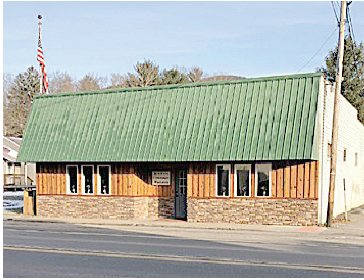
Rupert Community Building
