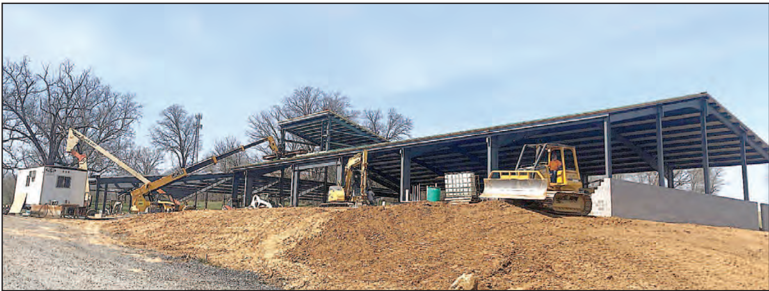
Construction crews can be seen excavating the pools.
