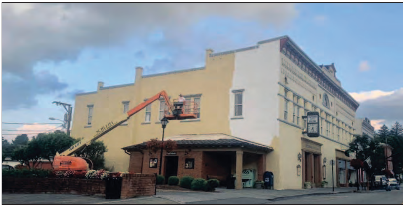
Schleiff Construction has been working hard on the tedious brick repointing and painting project for all of City Hall in downtown Lewisburg. Repointing is an essential part of the historic preservation of the building, as it prevents water damage and other issues that come with aging brick and mortar structures.
