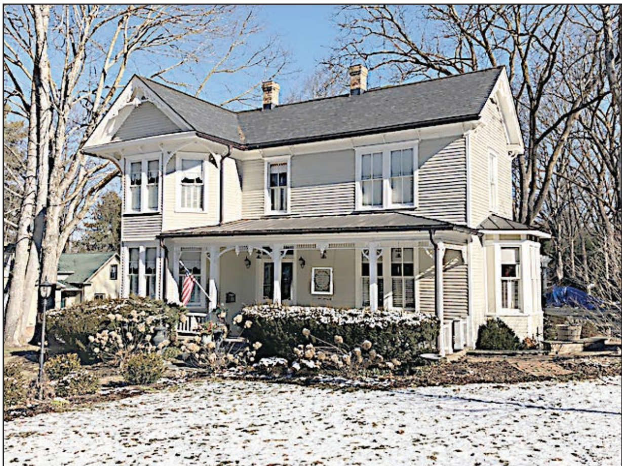
Dr. Jim and Jan DeHaven did a total restoration, inside and out, on this house in downtown Lewisburg, including raising the house to replace rotten parts and rebuilding the foundation. Schleiff Construction Co. was the contractor.
