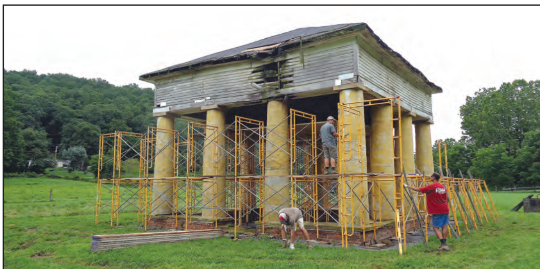
Before any work could begin, scaffolding was erected.
