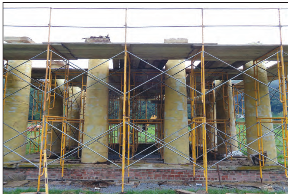
The roof was then removed (Cathy Bolt photo)
