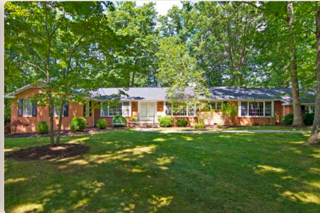
Lewisburg 22-1168 Well maintained custom brick ranch in Underwood Estates is close to all the amenities with 4 bedrooms, 2.5 baths, nice back brick patio, and more. $549,000
