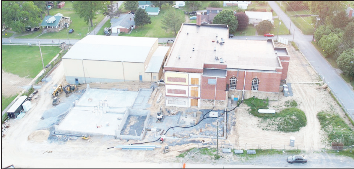
This overhead shot of the ongoing work to the future Alderson Elementary School (former community center) shows the extensive restoration, renovation, and construction efforts that are still ongoing. As of April, Greenbrier County Schools reports that they still plan to welcome students and faculty in 2024. (Photo by Wolfcreek Drone Photography)
