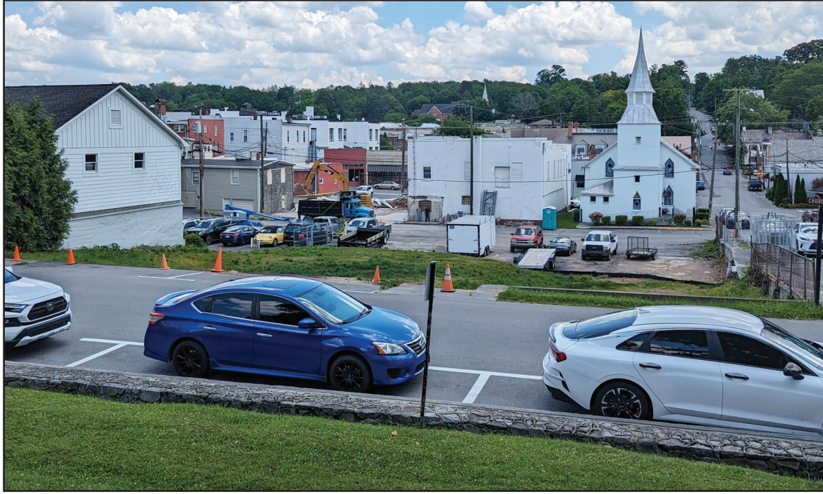
In the works for the old Seneca Health/True Value site are several townhouse/brownstone living quarters with garages, along with apartments, storefronts, and public parking. Final plans have yet to be nailed down, but the developers are working closely with the Historic Landmarks Commission, city officials, and local utility companies to finalize the details.
