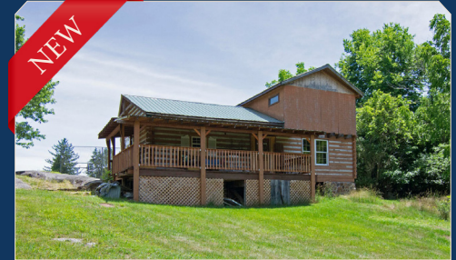
New Listing Union 23-744 Log home with 3 bedrooms, 2.5 baths ready to finish. Covered porch and outbuilding for garage or storage. $99,900
