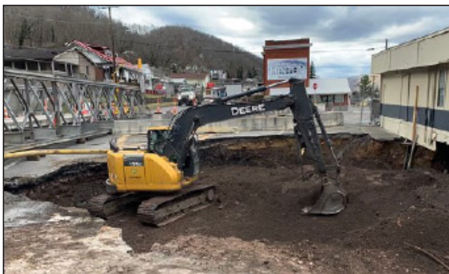
Temporary repair to large sinkhole that appeared in Hinton June 2022
