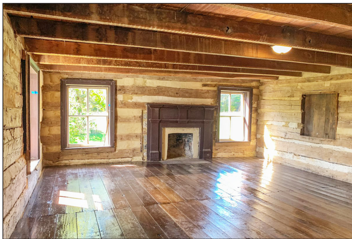
This room was once encased with plaster, including the ceiling.
