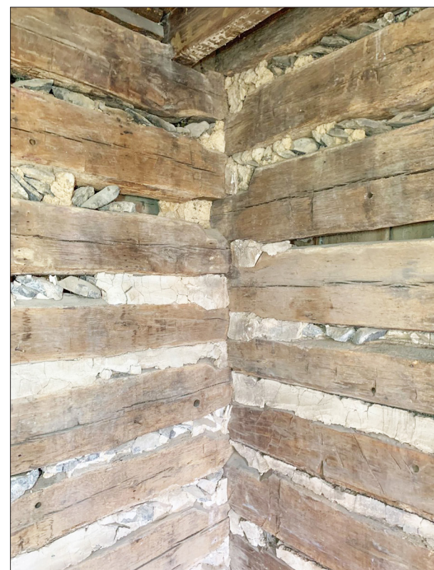
Rocks were revealed wedged in between the log walls of the home.
