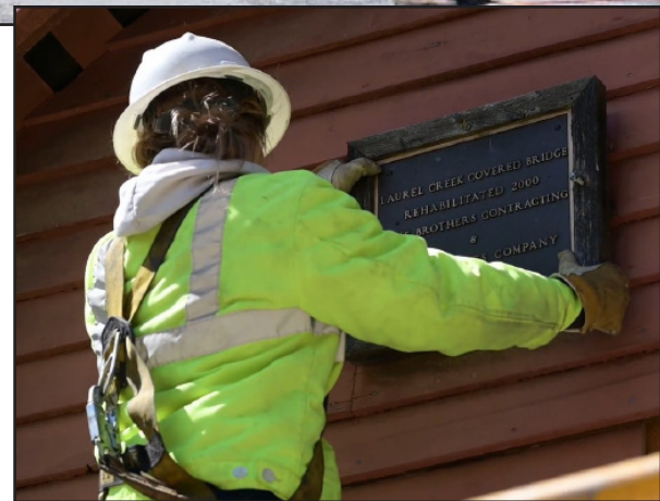
The informational plaque is reinstalled on the covered bridge.
