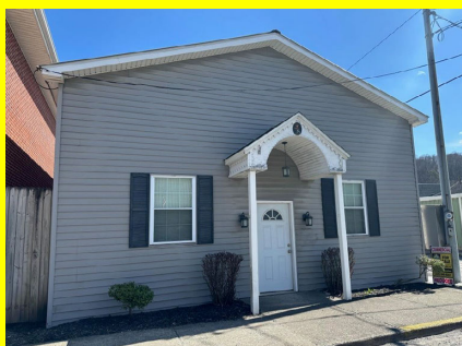
Rainelle $89,500 MLS #24-14 Updated commercial building with spacious offices and conference room. Liz Wickline (304) 646-8287
