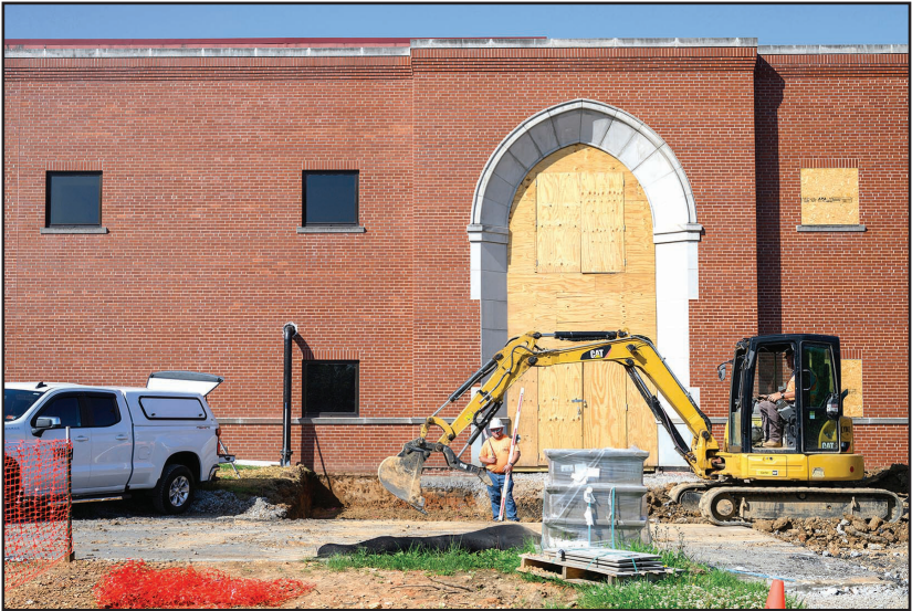
Science Building Construction
