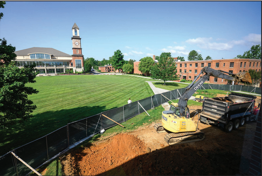
Science Building Construction
