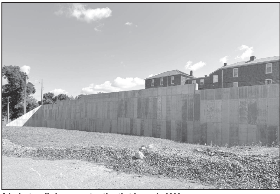
A look at preliminary construction that began in 2022.
