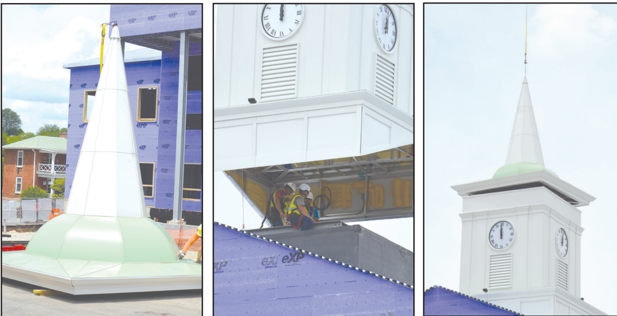
The Botetourt County Circuit Courthouse cupola was placed during a "topping off" ceremony last Friday afternoon in Fincastle. Here, three stages witnessed during the placement process.
