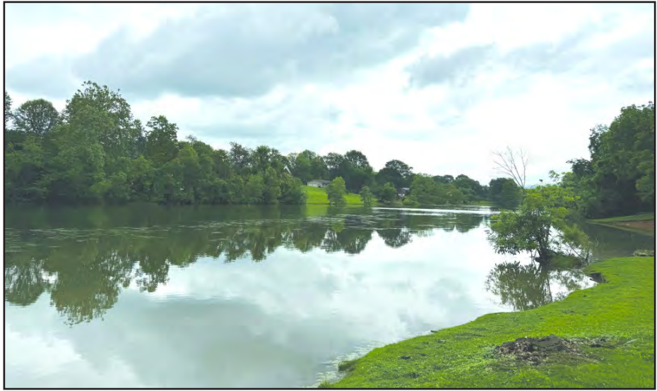
A recently completed engineering study of Orchard Lake in Daleville found the dam should be classified as high hazard because a failure could affect three downstream homes and nearby roads.
