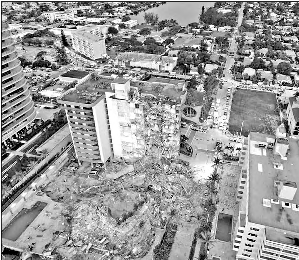
Part of a 12-story condominium that collapsed early Thursday morning in Miami-Dade County, Florida. Photo courtesy of the Miami-Dade Fire Rescue Department.
