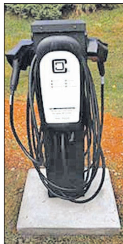
The electric charging station at the Montgomery County Government Center in Christiansburg has two charging ports, which allows two cars to charge at the same time.
