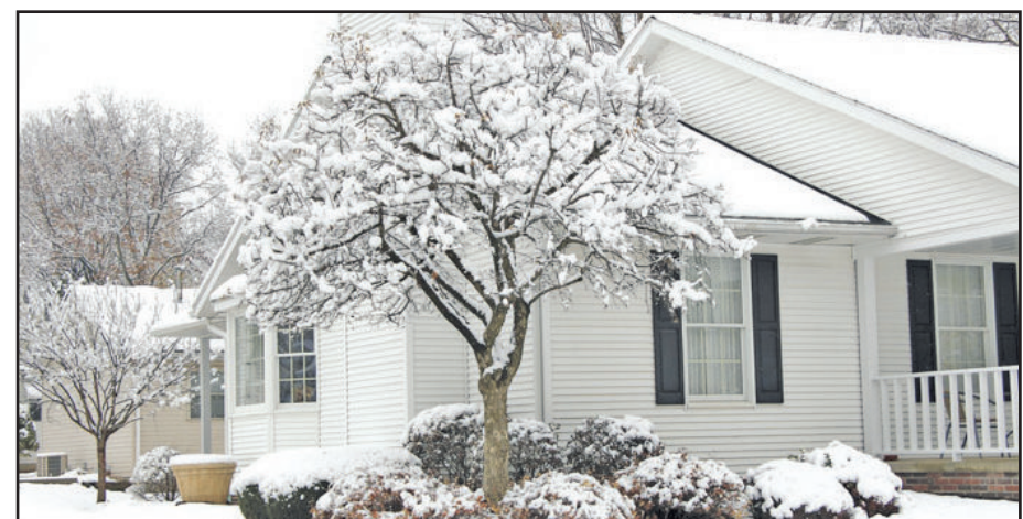
To prevent catastrophic damage to a home in the event of a sudden cold snap when the family is out of town, bump the thermostat into the 60s, not the 50s, let the faucets drip, and have a neighbor or friend check on the home periodically. Then remove any snow from the roof as soon as possible after returning home to prevent the snow from freezing.
