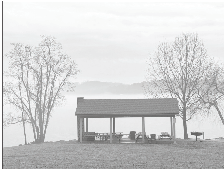
Claytor Lake State Park shelter after debris removal
