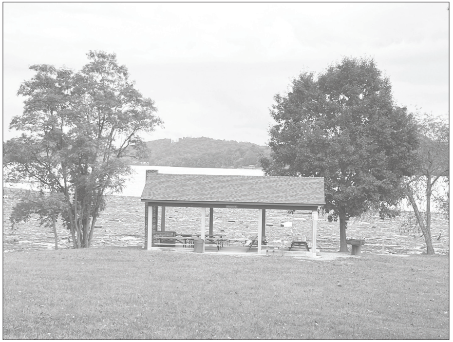
Claytor Lake State Park shelter before debris removal
