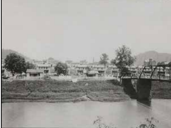
The old bridge and coal company houses are shown at Enterprise in 1921. Photo courtesy of Bobby Bice.
