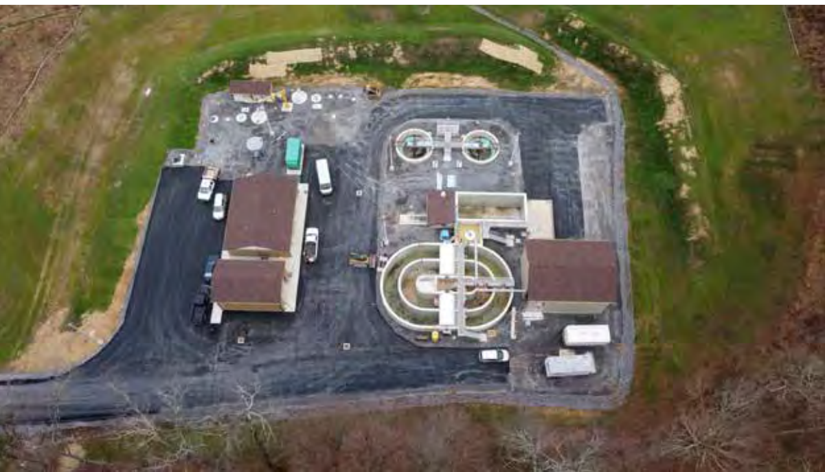
This aerial photo is of the Rt. 73 100,000 gallon per day Wastewater Treatment Plant. This plant services the Rt. 73 Corridor from the Auto Auction to Boothsville and was completed this year. Photo courtesy of The Thrasher Group
