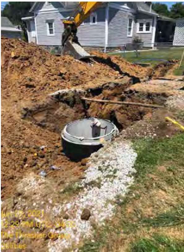
LOTS of dirt has been moved in the Enterprise area while sewer lines were put in place. The construction in that area is now 45% complete and should be finished by the beginning of 2022. Photo courtesy of The Thrasher Group.
