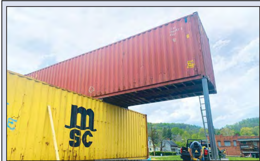
Work continues on a planned coffee shop made from containers in downtown Shinnston. Photo by Erin Beck.
