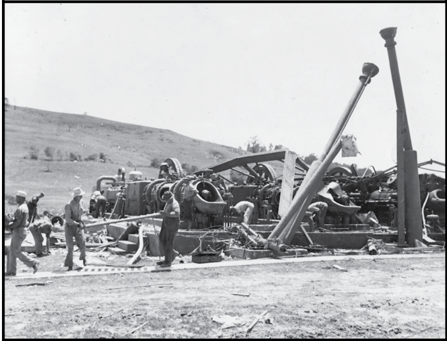
The June 23, 1944 tornado destroyed the Hope Natural Gas compressor station along Rt 73 in Bridgeport, although the remains, pictured, were replaced within six days. Photo courtesy of Bobby Bice.
