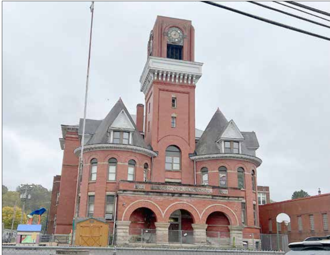
The Mannington Public School, built in 1902, demonstrates investment in education as the town developed its oil and gas industry.
