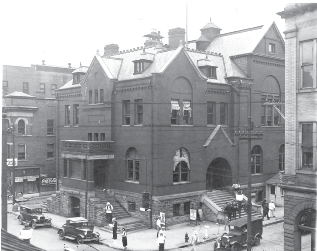
The old Federal Building, once located along West Pike Street in Clarksburg. Photo submitted by Bobby Bice.
