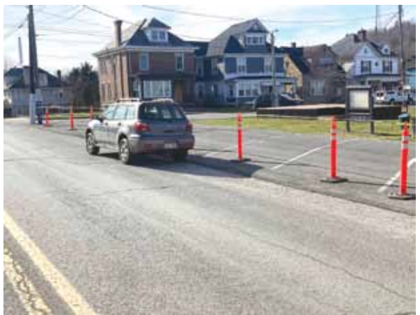
The parking lot was closed in mid-February after Division of Highways officials learned initially that it lacked a permit and upon further review, that work had paved over sidewalk access.
