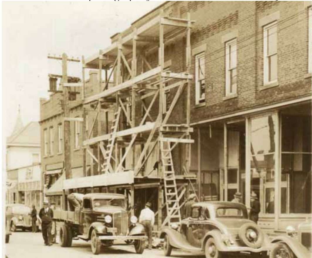
This 1930s view of the east side of the 400 block of Pike Street shows wooden scaffolding with a Leonard Riley Contracting Company pickup truck. Photo courtesy of Bobby Bice.
