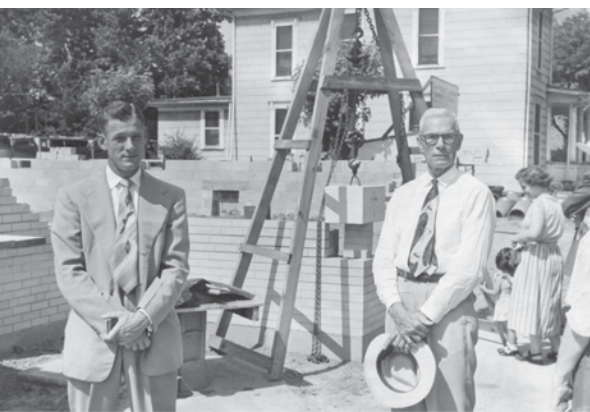
Laying a cornerstone and showing the depth of the Catholic Church tradition in Shinnston
