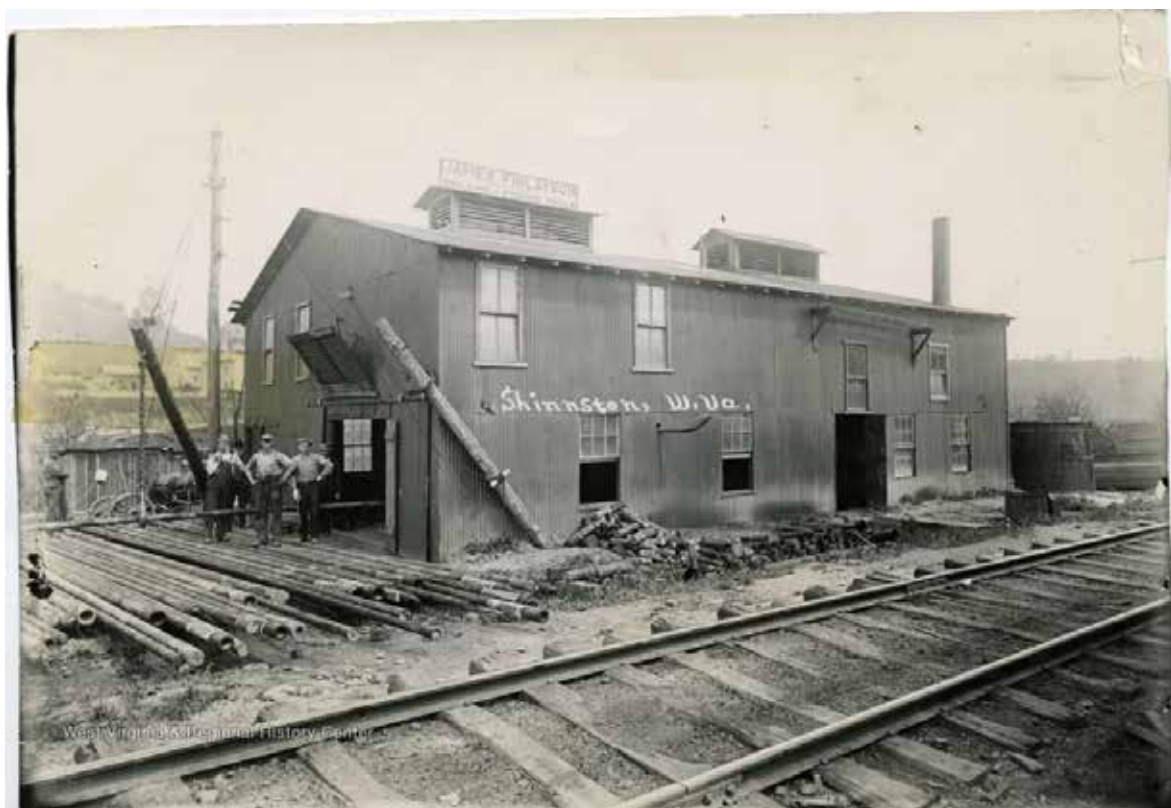
A group of men stand outside the James Finlayson Manufacturer of Drilling and Fishing Tools factory building in Shinnston, Harrison County, W. Va. No date given. Photo courtesy of West Virginia University
