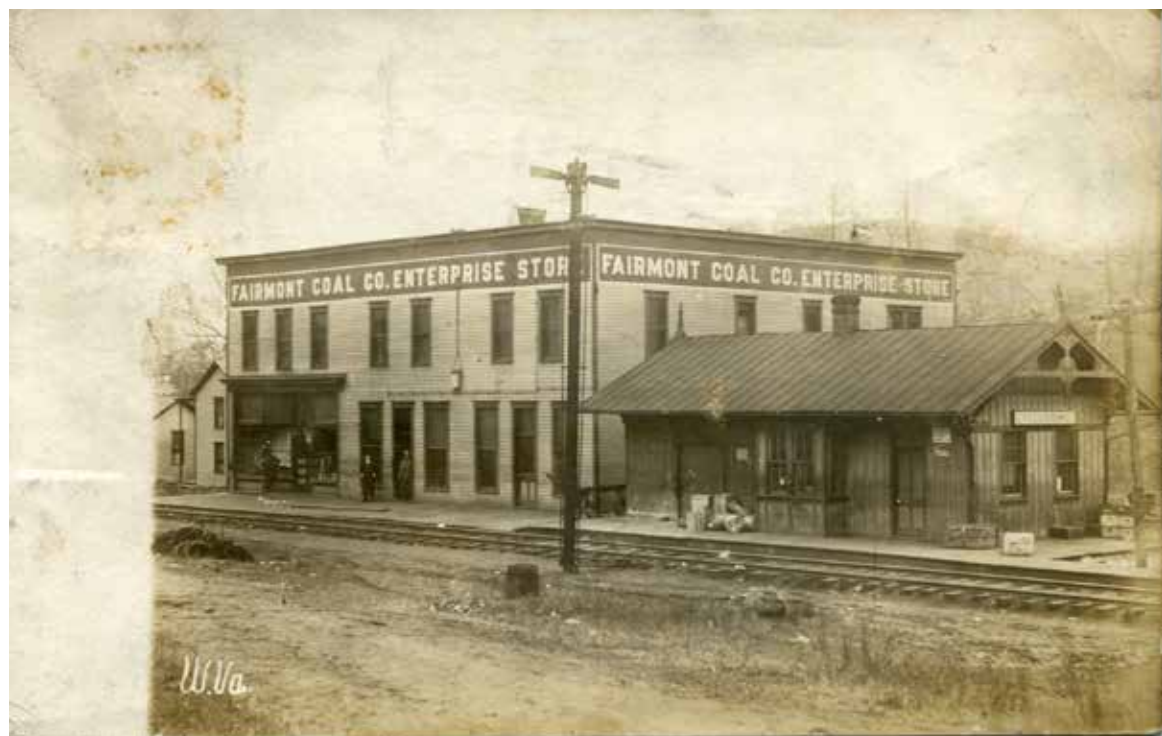
Shown are the Fairmont Coal Company Store and train depot at Enterprise. The store was built into the hillside & contained three stories; the basement level was accessible from the back side. The 3rd floor contained a meeting hall for several lodge organizations & had a separate outside entrance. A weight-operating elevator was also used in the building. Submitted by Bobby Bice
