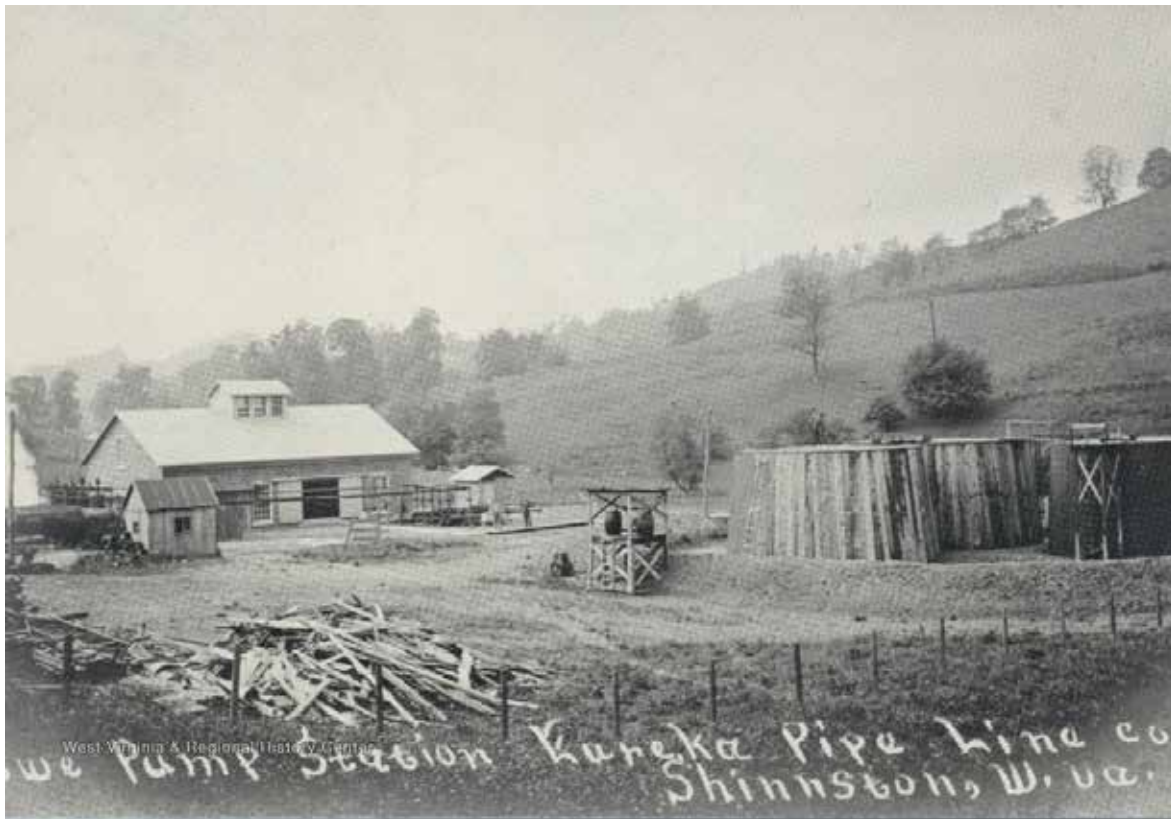
Pump station for Eureka Pipe Line Company near Shinnston, date unknown. Photo courtesy of West Virginia University
