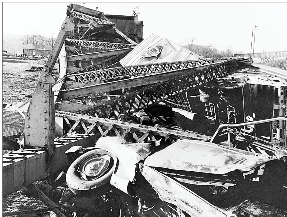
Dec. 15, 1967: The Silver Bridge at Point Pleasant collapsed, killing 46 people. The Silver Bridge was built by the American Bridge Company of Pittsburgh and opened to traffic on May 19, 1928. The accident led to the passage of legislation for a national bridge inspection and safety program.
