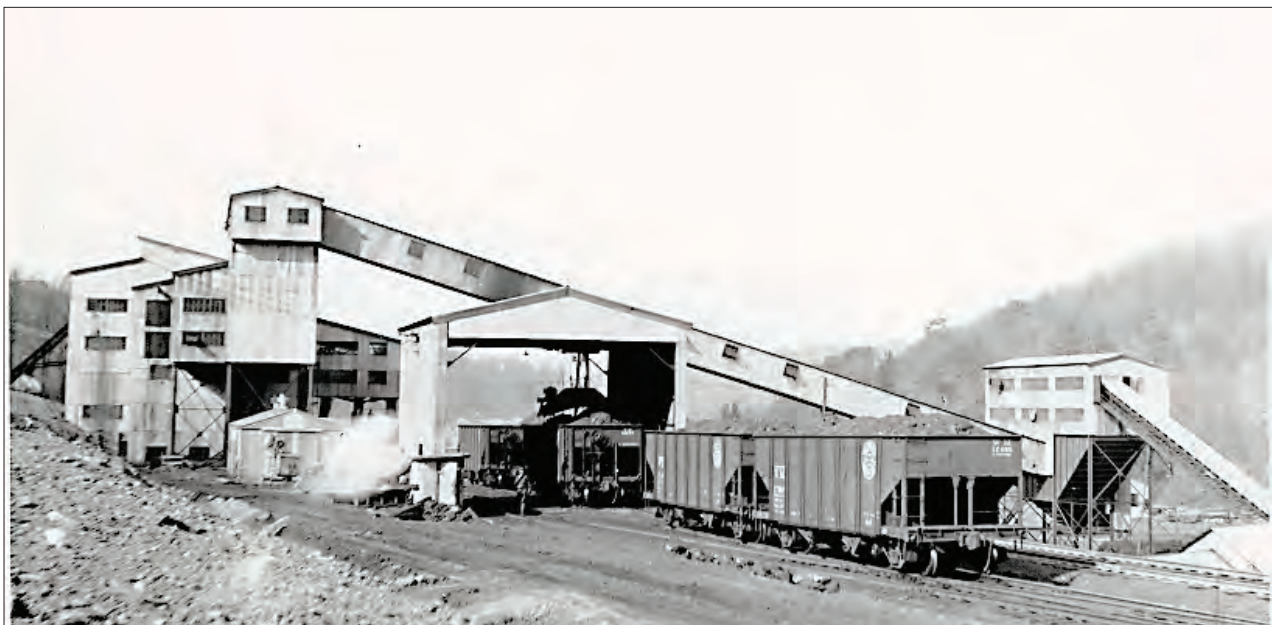
This photo was taken at the Bayard Washery on October 28, 1948. The photo shows raw coal arriving at the Bayard Washery. One hopper car is about to be dumped with the car "Shake Out". I do not have any further information on the process. Ideas, suggestions, comments, or items to share contact Tim Turner (304) 478-3389.
