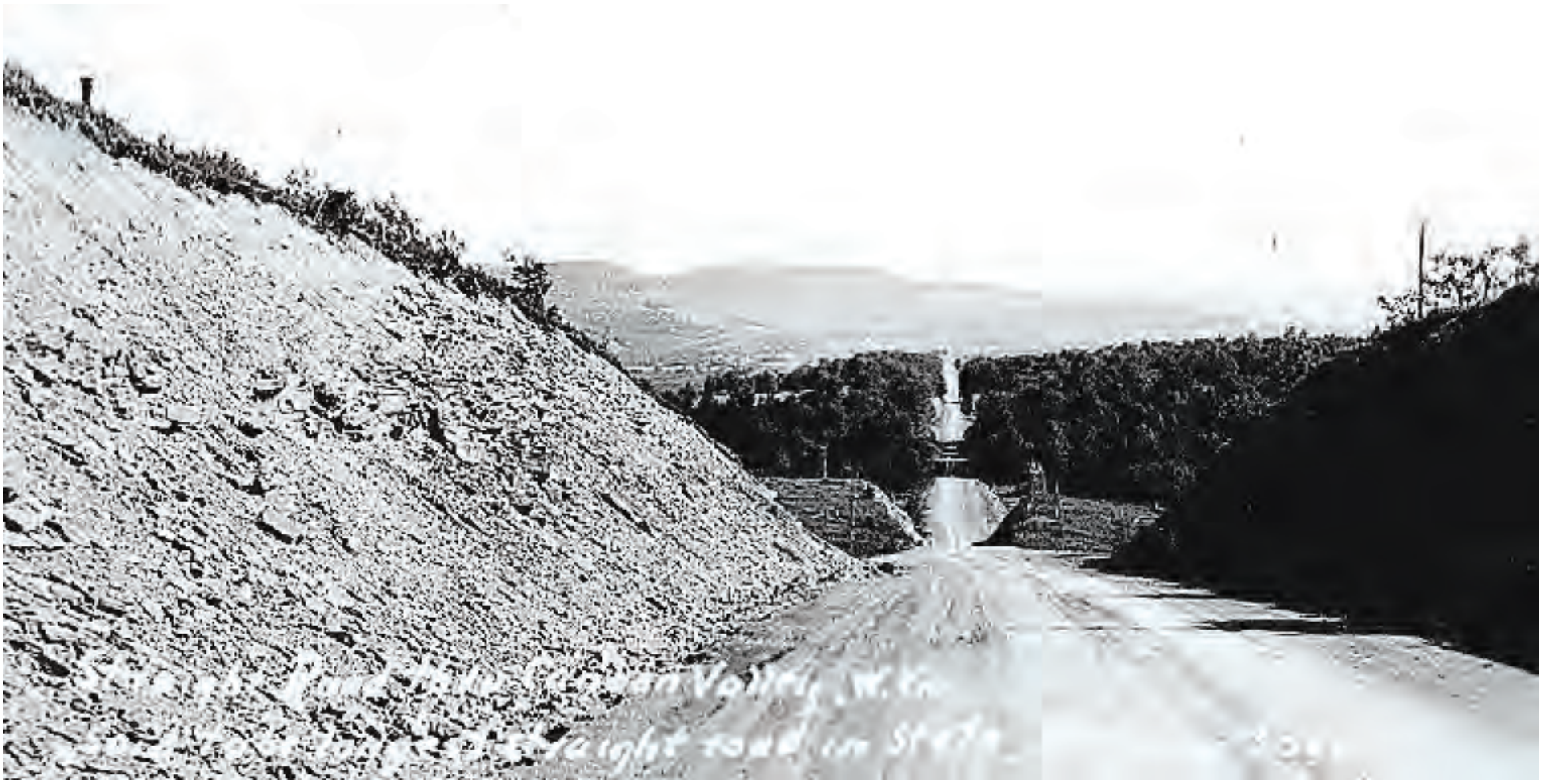
This is the straight road through Canaan Valley. At the time, it was said to be the longest straight road in the State. This road was kept above an elevation of 3000 feet so the dam (proposed Canaan Valley Dam) would not flood it when constructed. The road is known as Route 32 and the work began in 1932 and ended sometime in 1937. Many folks refer to this section of road as Canaan Straight. The road did not have a hard top surface in 1936 when the first school bus ran from the Valley to Davis. As you can see, the road is not paved in the photo. Ideas, suggestions, comments, items to share contact Tim Turner (304) 478-3389.
